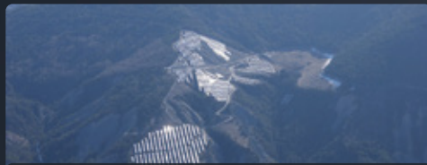
Photovoltaic Central – France
